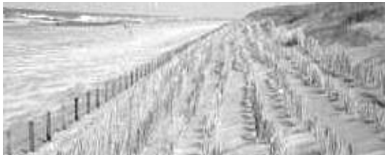
Figure 1: Traditional Dutch defence against the sea using bent-grass.
